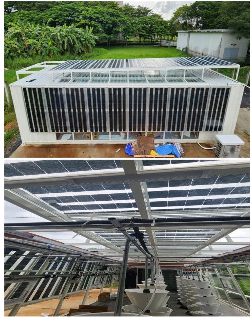
Fig. 1. Sprout ginseng cultivation system using natural light distributed solar module (Top: outside, Bottom: inside)
