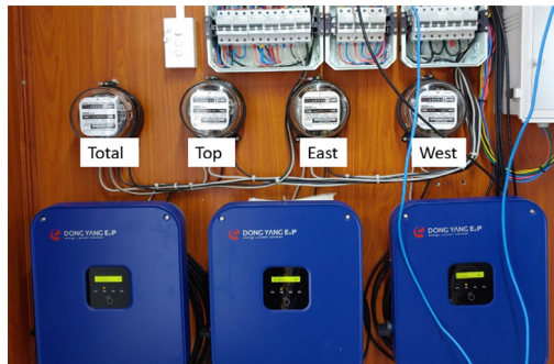
Fig. 2. Installation of 3 kW inverter and power meter
